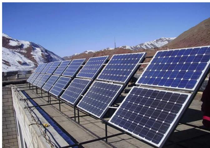
**Figure 3:** mono-crystalline silicon solar panels [6]
