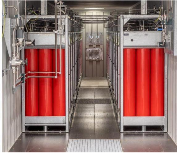
Figure 17: Inside a hydrogen storage container [40]
